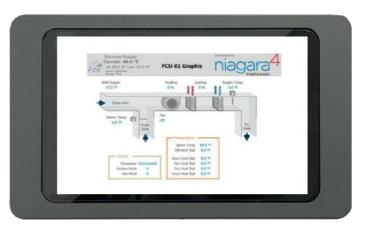
HIGH QUALITY, PANEL OR WALL-MOUNTED, TOUCH SCREEN DISPLAY. COMPATIBLE WITH ALL MODERN WEB-SERVING BMS CONTROLLERS.
